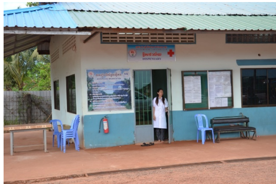
Construction and maintenance of a small clinic and pharmacy
